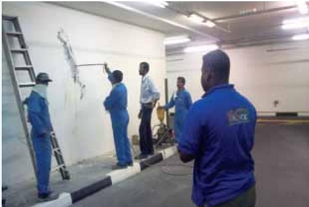
Crack and Leak Injection | Basement of Head Office Buiding | National Bank of Abu Dhabi
